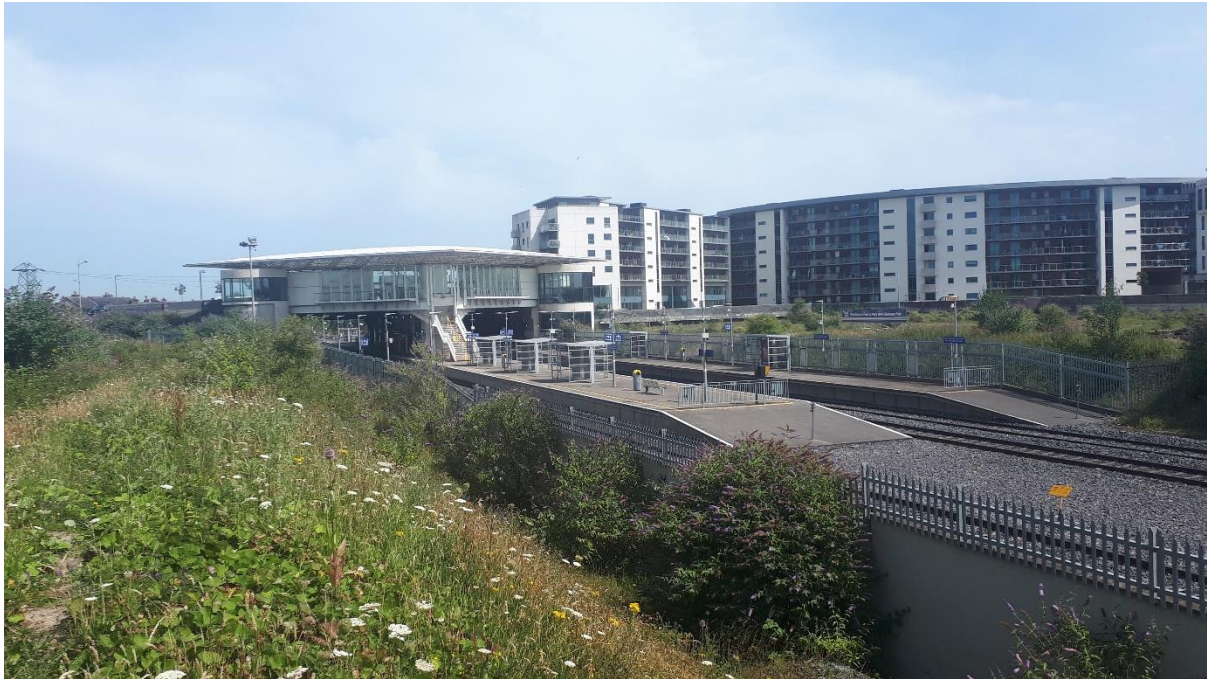
Figure 10.5 View of the southern boundary, railway cutting and Cherry Orchard railway station, with the Concert and Crescent buildings in the background. Note the pylon on the left, located within the development site.
