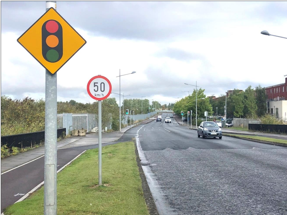
Figure 14.3 Park West Avenue looking north from the bridge over the railway.
